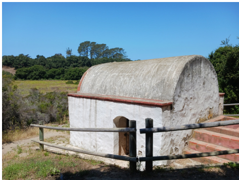
Photo: Springhouse fed by a separate spring, the springhouse features a settling box and interior tank. Water is channeled downhill from the springhouse to the aqueduct. Photo by Doug Bradley.
