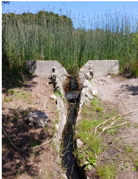
Photo: Pond outlet. Purísima's aqueduct system begins at the northern pond, located just off the Las Zanjias service road. Satellite imagery suggests a storage size of approximately 0.15 acre feet. Photo by Doug Bradley.
