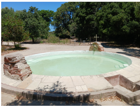
Photo: Indian lavandería used for both bathing and washing; the outlet box (right foreground) channeled water to a separate drainage. This cistern held about 12,000 gallons. Photo by Doug Bradley.
