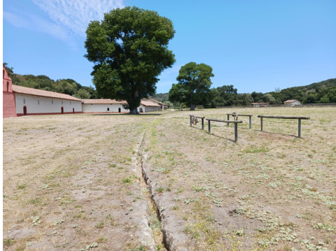
Photo: South end of aqueduct. This is the southern-most terminus of Purísima's aqueduct system and final destination for graywater leaving the central mission grounds. Photo by Doug Bradley..
