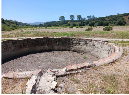
Photo: Large upper cistern looking south from its inlet toward the mission grounds. The aqueduct can be seen in the distance on the left side. This is Purísima's largest cistern (42,000 gallons) and is the first stop for pond water on its journey to the mission. Photo by Doug Bradley.
