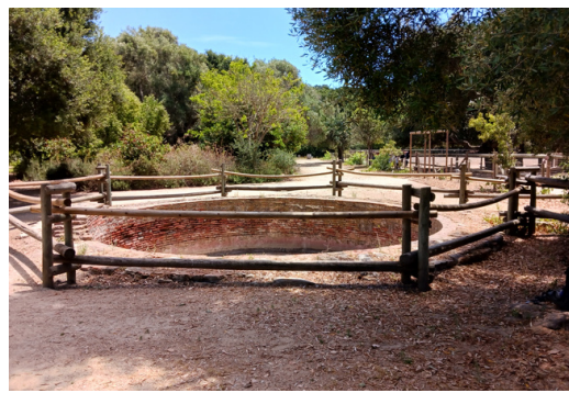
Photo: Central cistern” — The central cistern held graywater from the central lavandería only a few meters north. Water was stored for crop irrigation near the church. Photo by Doug Bradley.
